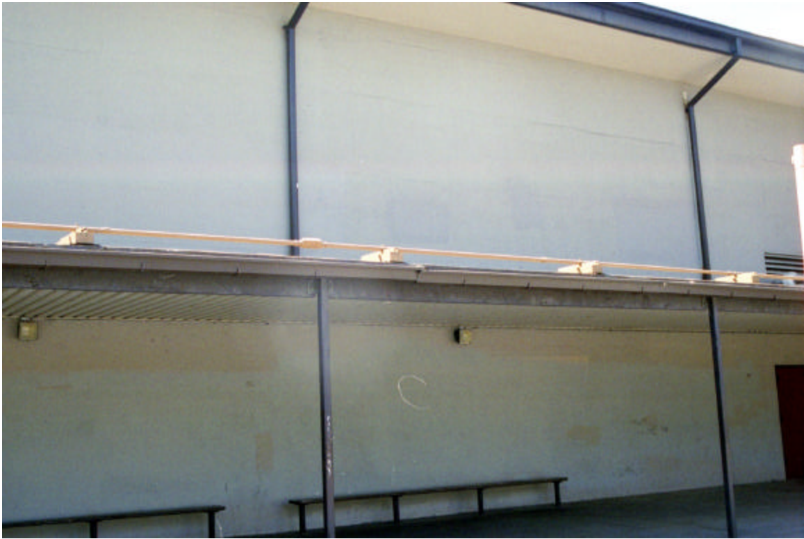
FIGURE 8: GYMNASIUM BUILDING, NORTH ELEVATION
