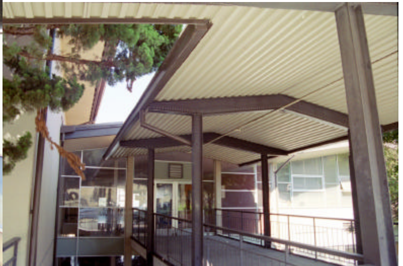
FIGURE 5: ACADEMIC BUILDING, EAST ENTRANCE
