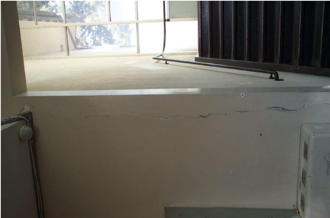
FIGURE 16: ACADEMIC BUILDING, END CONCRETE/STUD WALL SEPARATION
