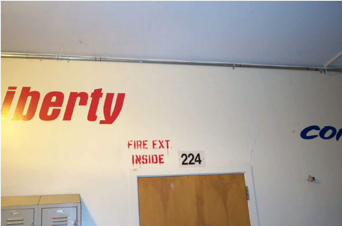
FIGURE 17: ACADEMIC BUILDING, CENTER STUD WALL LINTEL PLASTER CRACKS
